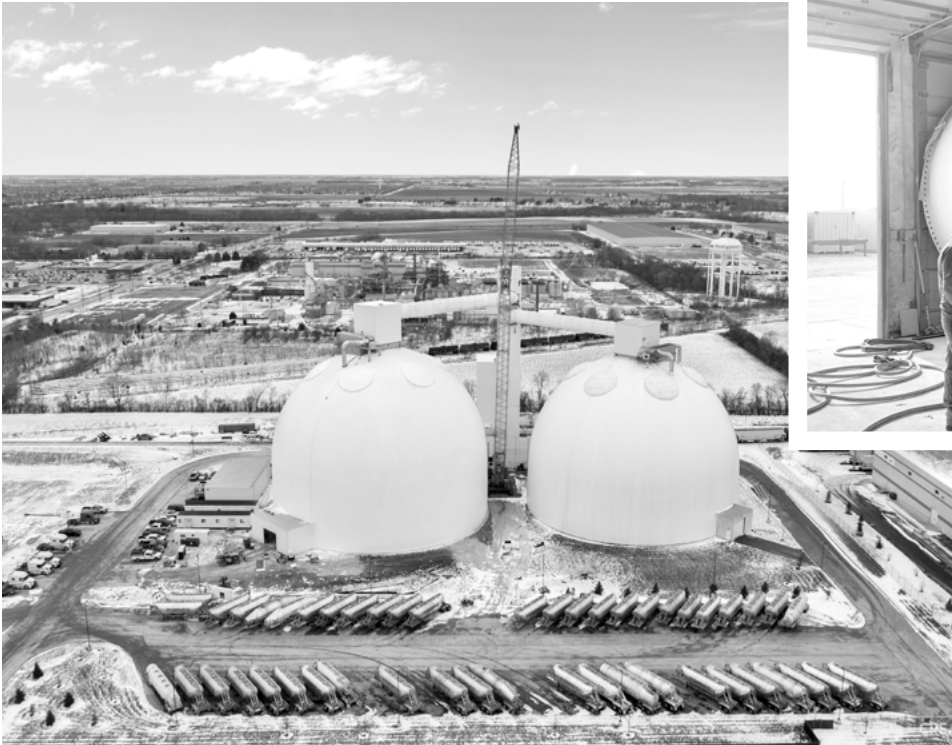
Dome Technology is building a second dome, pictured on the left, for American Crystal Sugar in Montgomery, Illinois, USA. Above: The tube gallery connecting the domes was fabricated at the Dome Technology shop in Idaho Falls, Idaho, USA.
