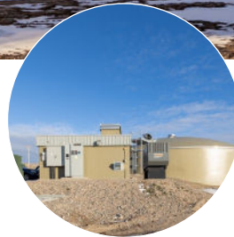
Dome Technology also built the adjacent pump house.
