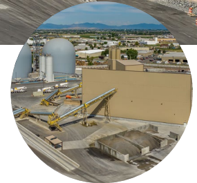
Fly ash and cement from the DomeSilos can be conveyed to the ready-mix plant, the tan structure at right.
