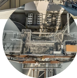
Fly ash or cement fills either dome from the rail-unloading building.
