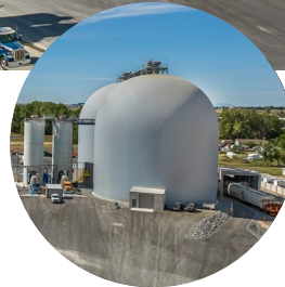
Trains deliver product, right, and cement is transported out by truck, left.
