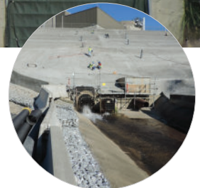
With the slope stabilized, water is directed in such a way that the nuclear station is better protected.
