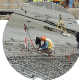
Rebar placed on the hillside adds strength to the finished concrete.
