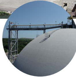
The DomeSilo is 171.5 feet tall and 165 feet in diameter, maximizing storage on a small footprint.
