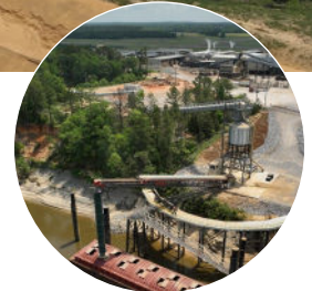
Pellets are later conveyed 1,000 feet to be loaded on barges.
