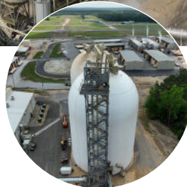
A bucket elevator conveys pellets into the first dome.
